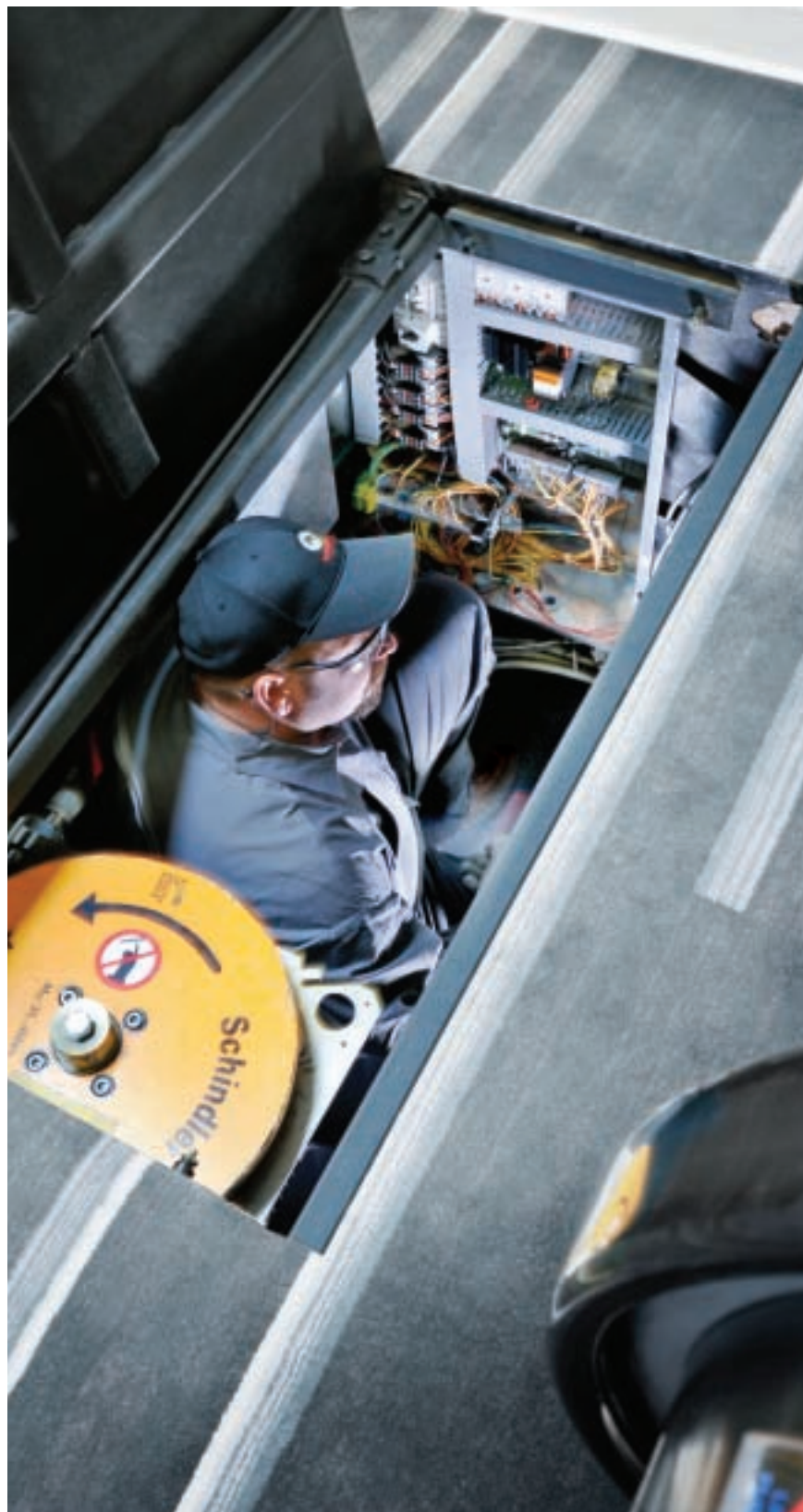
A Schindler technician makes final adjustments to an escalator’s new solid state controller.
