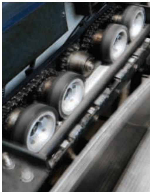
Photo above: Schindler technicians remove old handrail. Photo right: The new handrail drive assembly. Photo far right: The new handrail speed monitor.
